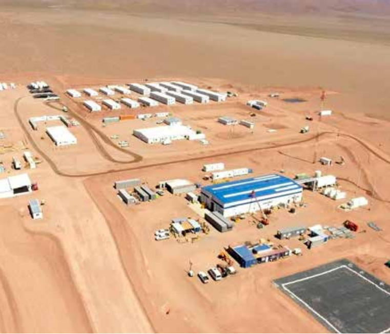
Lithium exploitation plant in Salta, Argentina. Image: mineriyadesarrollo.com
